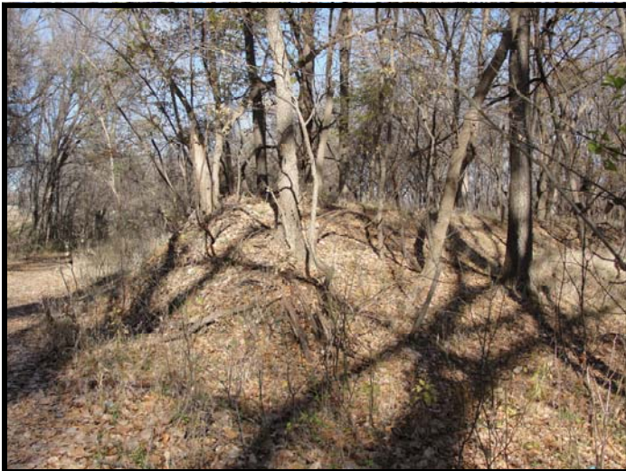
Traveling on Frank Phillips Blvd. during the winter months, when the foliage is sleeping, the Interurban embankment is visible on the south side of the road. The Interurban tracks were constructed on this embankment which was constructed of cast-off materials from the smelter operations of the Lanyon-Starr, Bartlesville Zinc and National Zinc Companies.
