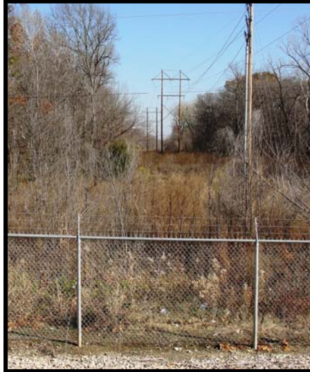
Looking east from PSO, through the break in the trees and over the hill is the support system for the Interurban Bridge
