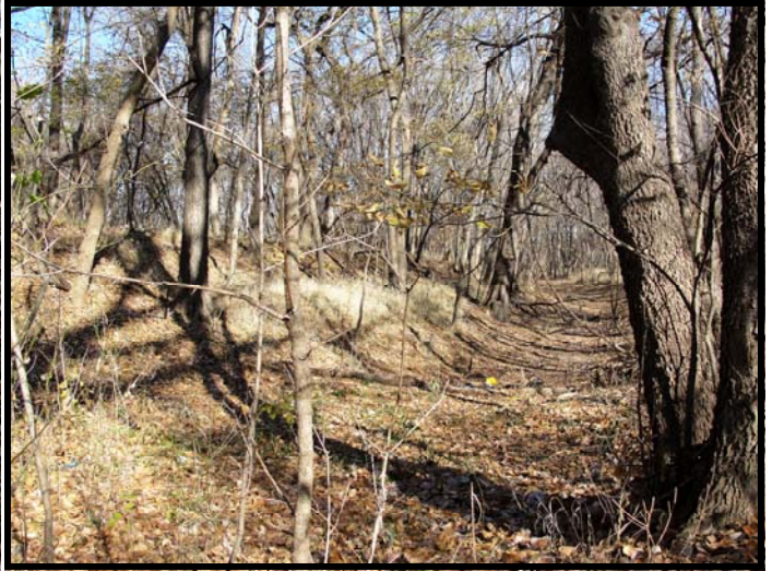
Traveling on Frank Phillips Blvd. during the winter months, when the foliage is sleeping, the Interurban embankment is visible on the south side of the road. The Interurban tracks were constructed on this embankment which was constructed of cast-off materials from the smelter operations of the Lanyon-Starr, Bartlesville Zinc and National Zinc Companies.
