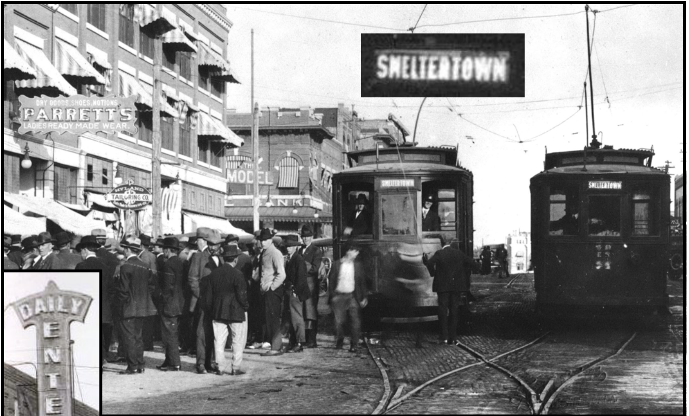
Third Street switch/pass (later Frank Phillips Blvd.) in front of Parretts Dry Goods with the Model Clothier (later May Brother's Clothing) in the background. This switch allowed the Interurban cars to pass in route to and from Smelertown (National Zinc, Bartlesville Zinc and Lanyon-Star Smelting Company—at that time the largest smelting company in the world).
