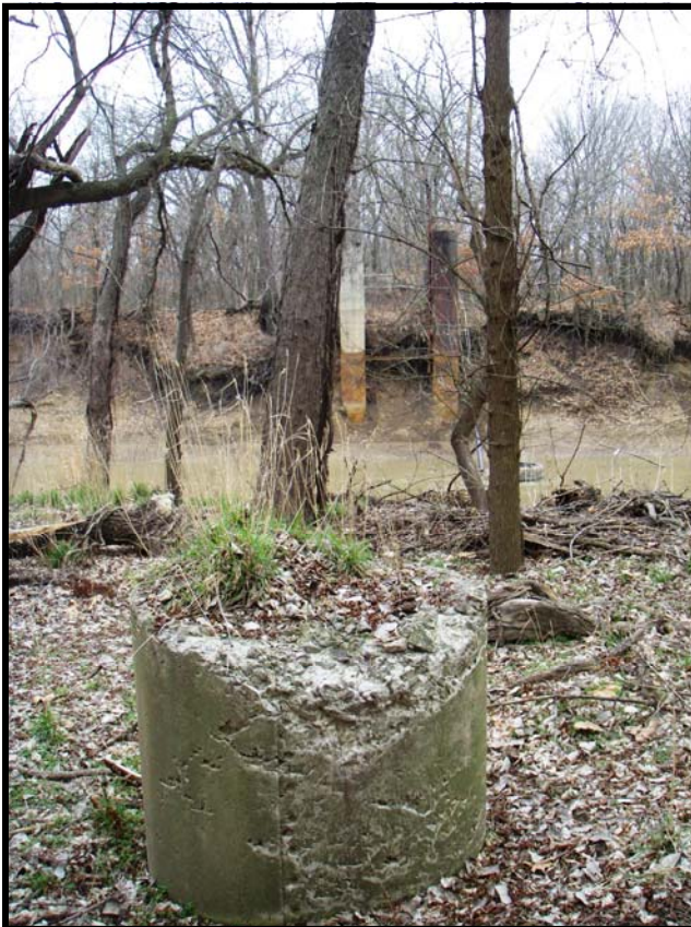
East of the Caney River and south of the Frank Phillips bridge, concrete support bases remain in wooded areas.
