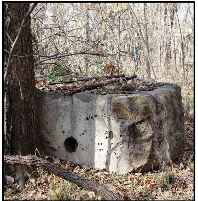
Many massive concrete supports remain in the wooded areas. This photo was taken south of Frank Phillips Blvd. just before the Caney River bridge and follows the line of travel from the Interurban terminal east to the Tuxedo area and the north to Dewey.
