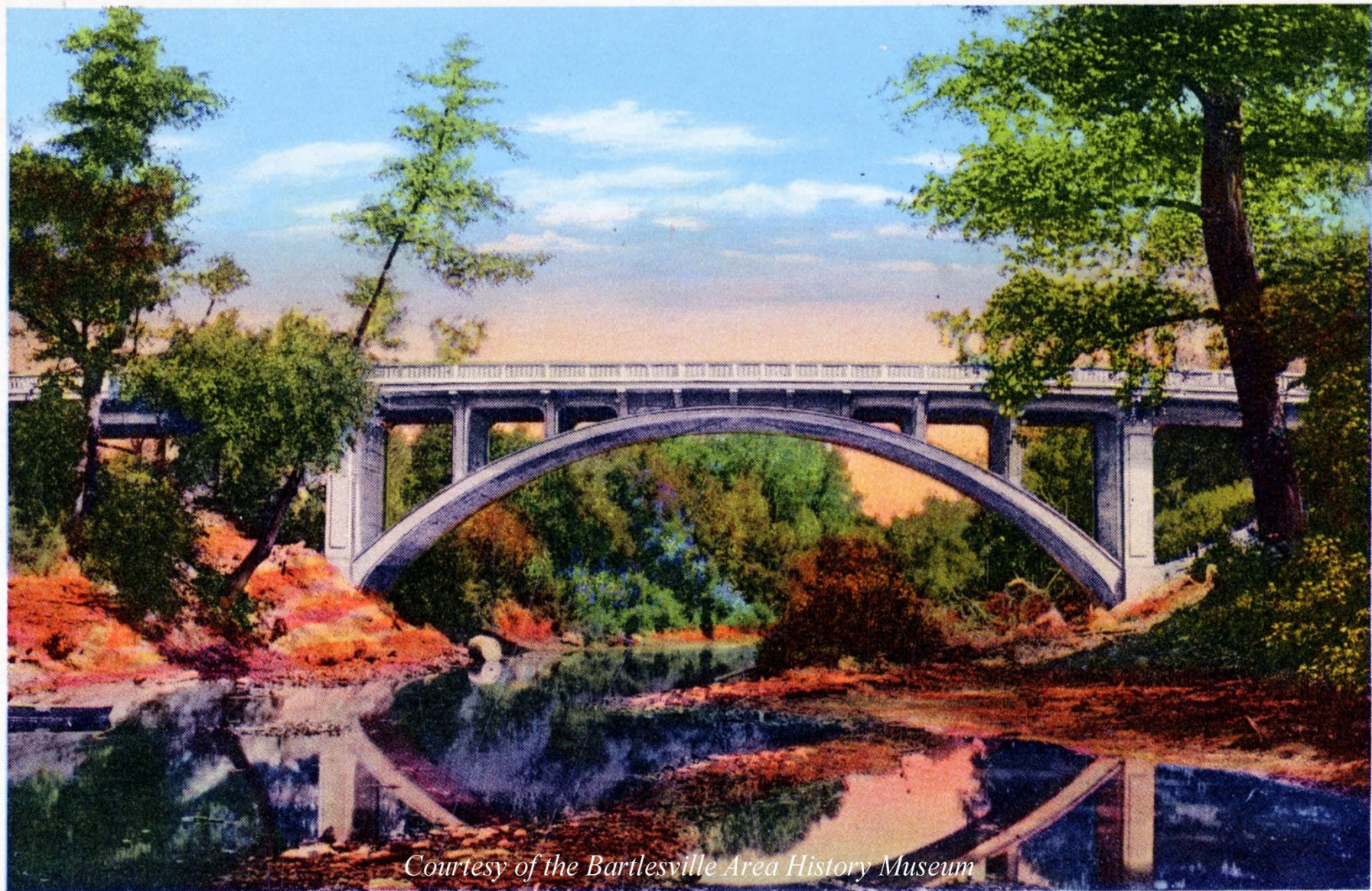
Memorial Bridge, Bartlesville, Okla.
