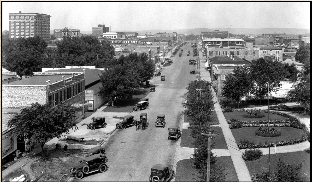
Bartlesville between 1922 and 1925. This photo was taken from the Washington County Courthouse looking to the west showing the 400 block of East Third Street. On the right is the lawn of the Washington County Memorial Hospital built in 1922. To the left is a Chevrolet dealer facing north and the O.B. Toalson Lumber Company at the corner of Cherokee Avenue and Third Street.
