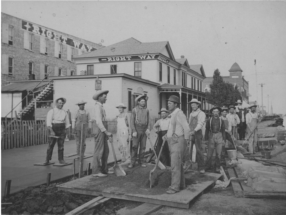
Laying concrete walk along Right Way Hotel on north side of Third Street in 1905
