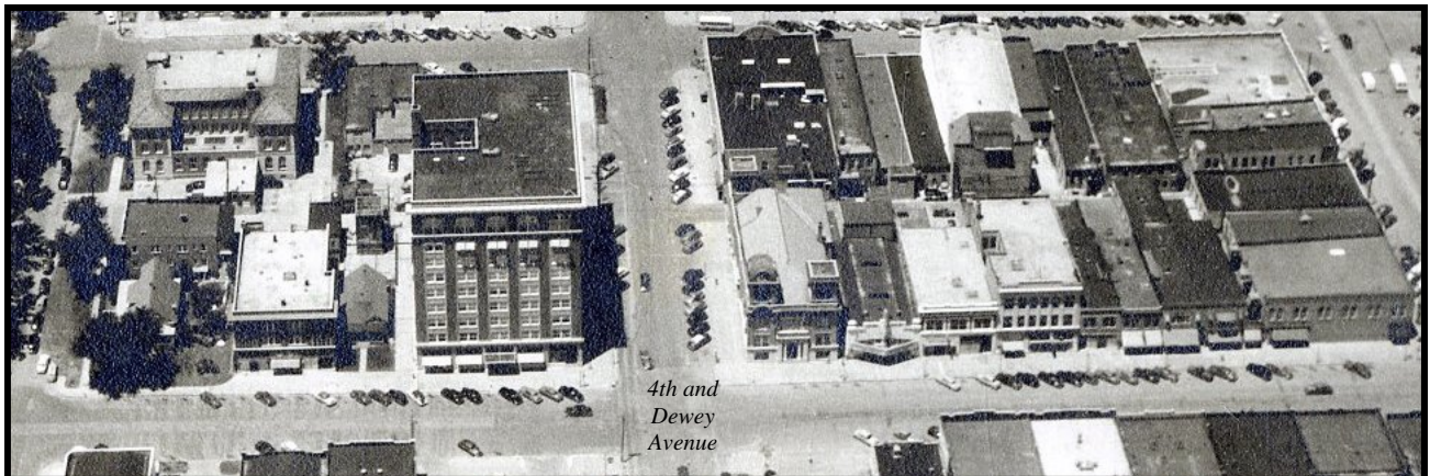
Left above shows the Aurora Building nestled among homes in the 400 block of S. Dewey Ave. with the Masonic Building at the corner of 4th Street and Dewey Avenue.
